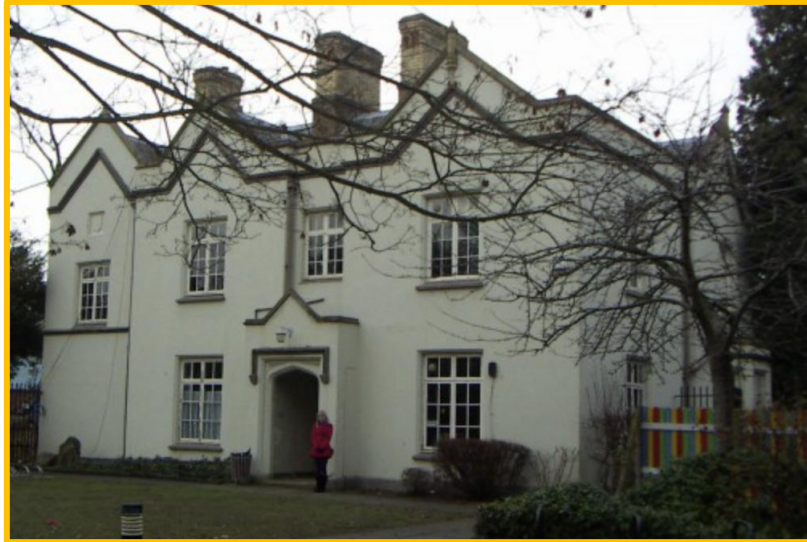
The Old Quorn Vicarage a nursery school in modern times It was built on Glebe lands
