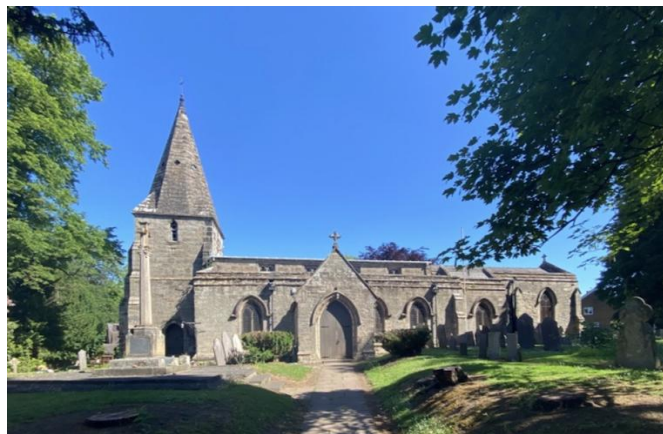
Church of St. Michael Ravenstone
